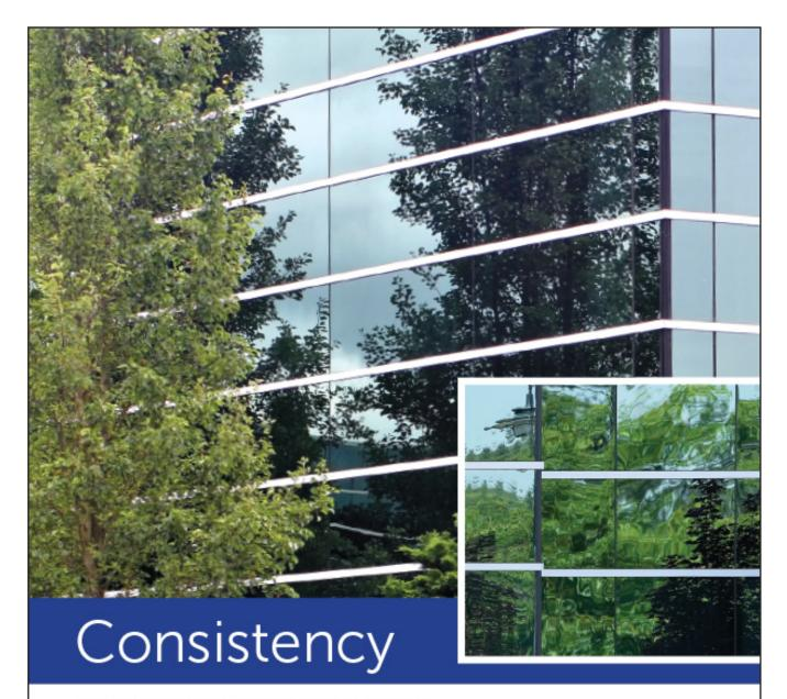
All glass that is subjected to the heat treating process will have some degree of distortion. Poor control of this process can increase distortion significantly (see inset).
